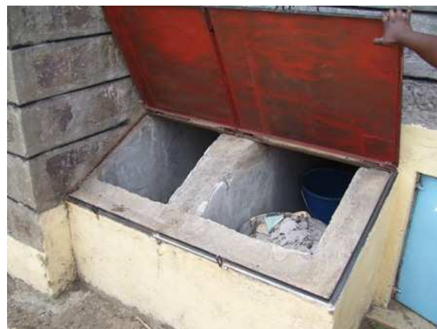
Fig.13: Containers are placed in the solar drier of the double vault compartment
