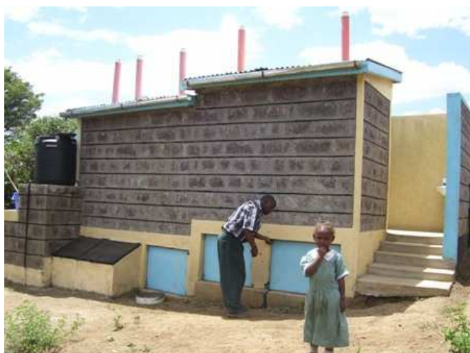
Fig. 11: The rear of the UDDT showing the single vaults and the solar drier for the double vault
