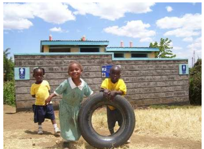
Fig.3: The front view of the UDDT with the men/boys side on the left and the ladies/girls on the right (source: C.Rieck 2008).
