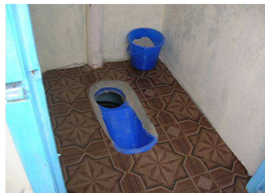
Fig. 6: Inside the single vault toilet at the church showing the urine diversion pedestal and a container of ash.
