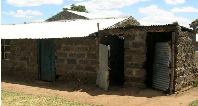
Fig. 4: Existing pit latrines
