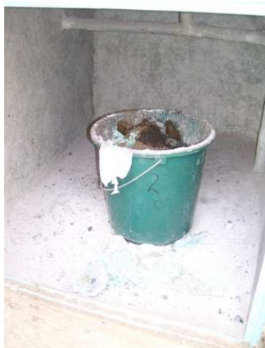
Fig. 10: 20 liter container in a single vault
